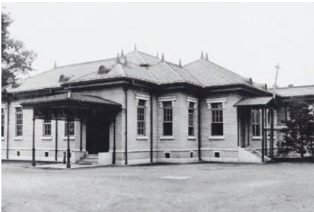
Former Mitsui Bunko exterior (property of Mitsui Bunko)
